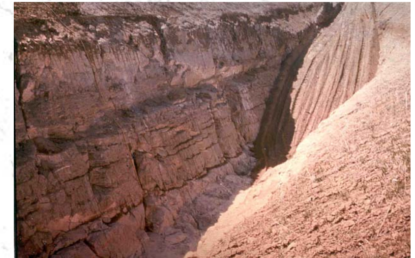
Teton Dam Core Trench and Foundation, Idaho, USA from USBR
