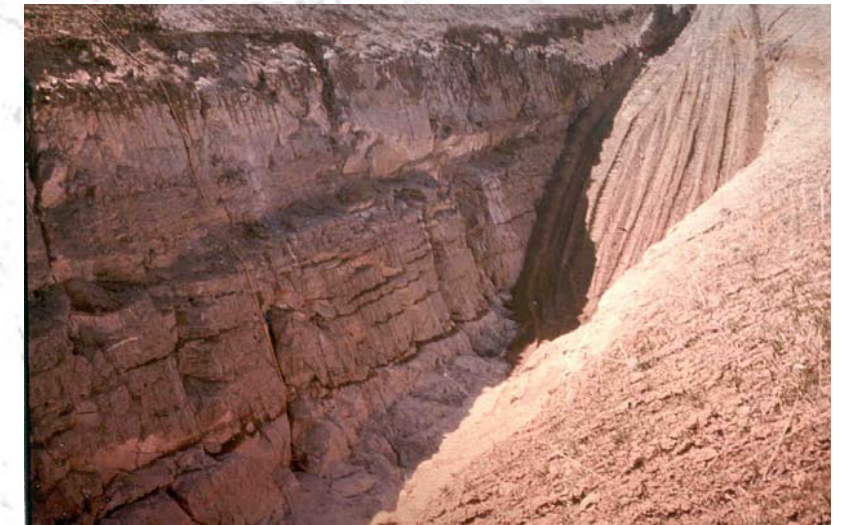
Teton Dam Core Trench and Foundation, Idaho, USA from USBR
